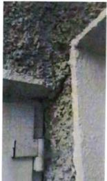
A Flavour of the internal and external damage, caused by constant Blasting. No one Blast may be above the permitted level however on a weekly basis the constant Blasting caused damage over time
